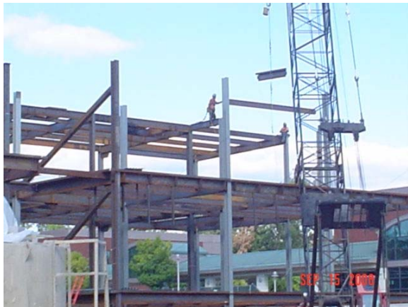
Figure 1, Steel Erection via Lattice Boom Crane
