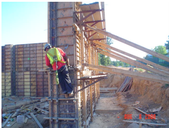
Figure 3, Support and forming of north retaining wall
